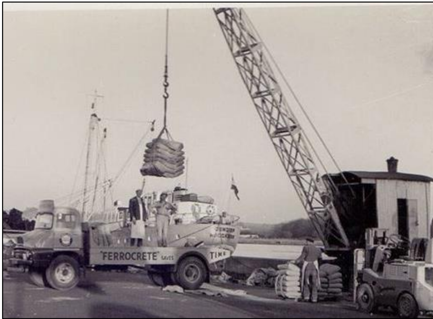
Cement lorry being loaded late 1960's
